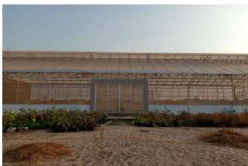
PHOTO 7: GREEN HOUSE, PLANT PROTECTION CENTRE, DEPARTMENT OF AGRICULTURE MINISTRY OF AGRICULTURE & FORESTRY
